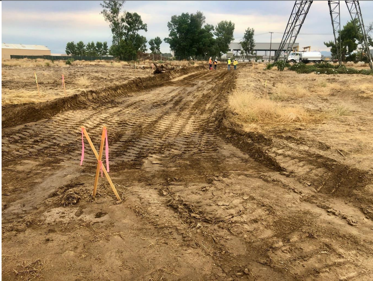
Photo 4 – Road recompaction work. Photo facing south
